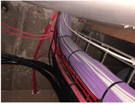
Electrical riser fire stopping inadequate
