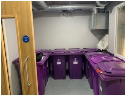
Waste stored internally
